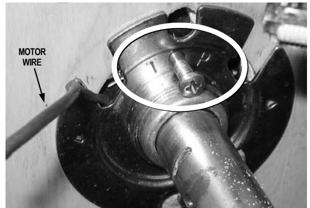
FIG. 12: INSIDE ROSE PLATE INSTALLATION
