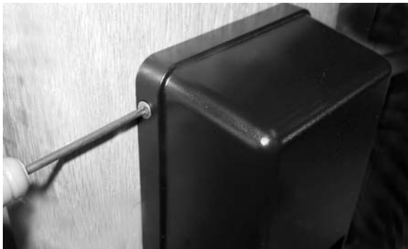
FIG. 16: SECURE TOP OF INSIDE HOUSING
